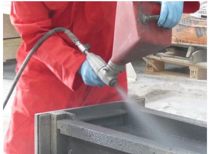
Application of Facing Coat using hopper gun
